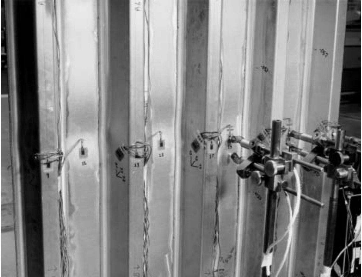
(a) Buckle at centerline of panel.
