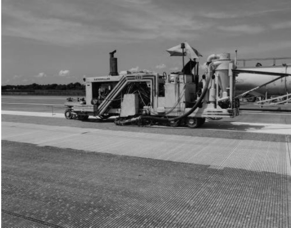
Figure 16. Large diamond-blade-grinding machine.
