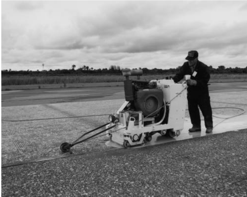
Figure 14. Diamond-blade-grinding machine.
