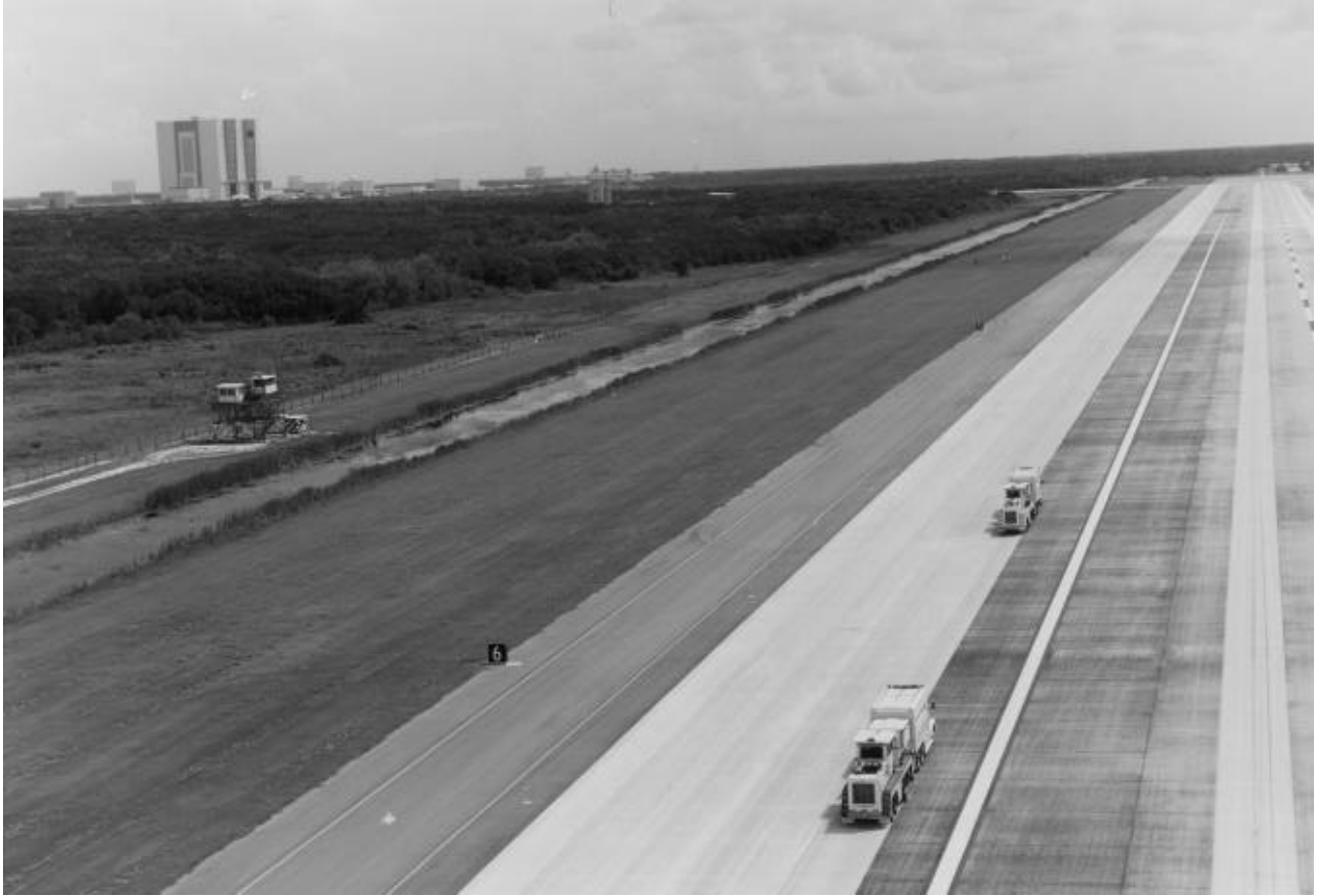
Figure 31. View of Skidabrader™ machines modifying entire SLF runway.
